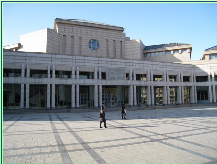
Peking University Centennial Memorial Hall, Beijing, China
